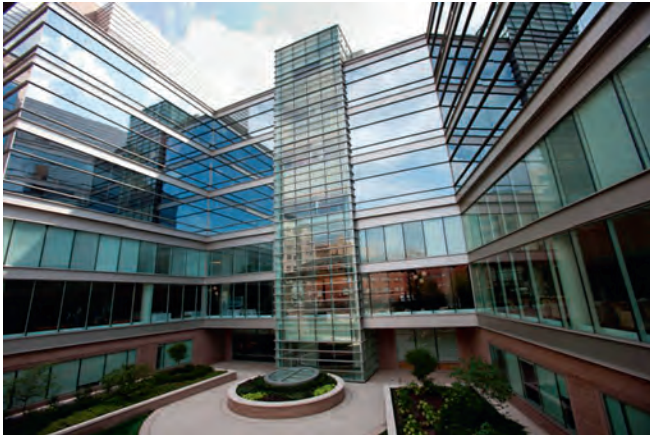
North Carolina Cancer Hospital, Chapel Hill, N.C.
